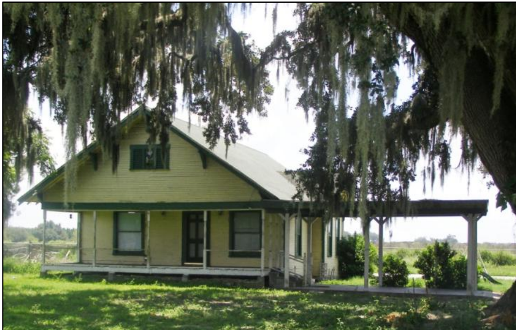
Photo 6-11. The north and west elevations of the Frame Vernacular style residence at 601 W SR 60 (8HI11919).
