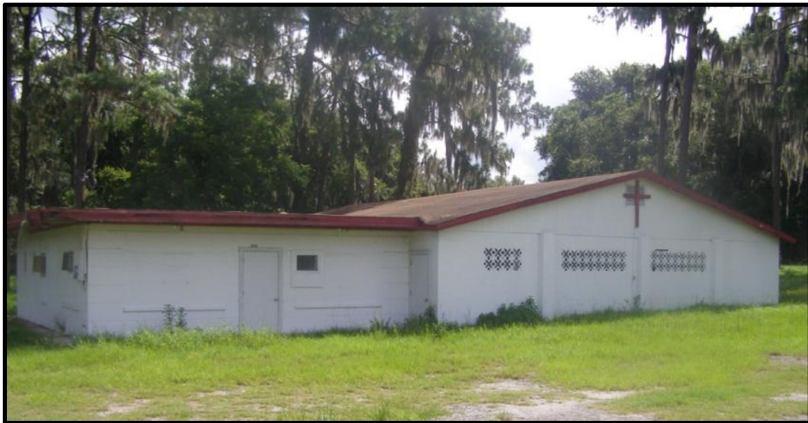
Photo 6-15. The west and south elevations of the Masonry Vernacular style church at 2414 E SR 60 (8HI11934).
