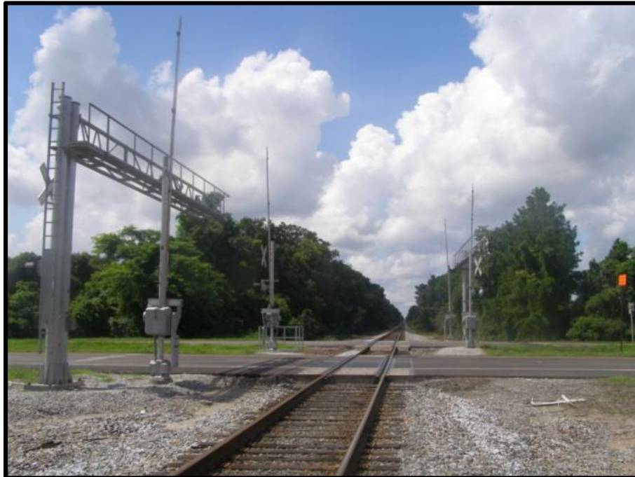
Photo 6-9. The CSX Railroad (8HI11888) where it traverses SR 60 (8HI11991).
