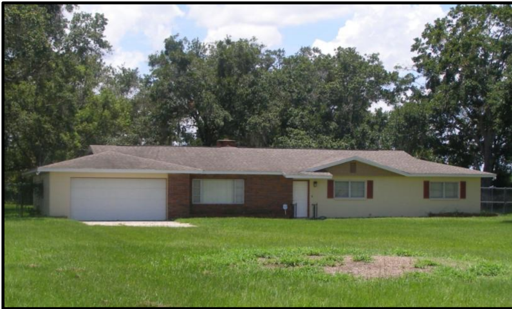
Photo 6-17. The north elevation of the Ranch style residence at 303 W SR 60 (8HI11920).
