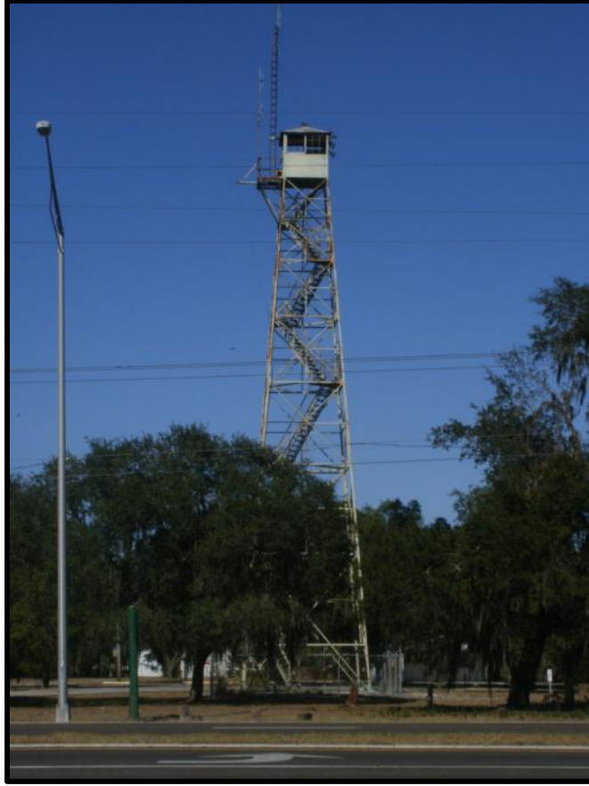
Photo 6-6. The south elevation of the Valrico Fire Tower (8HI3880).
