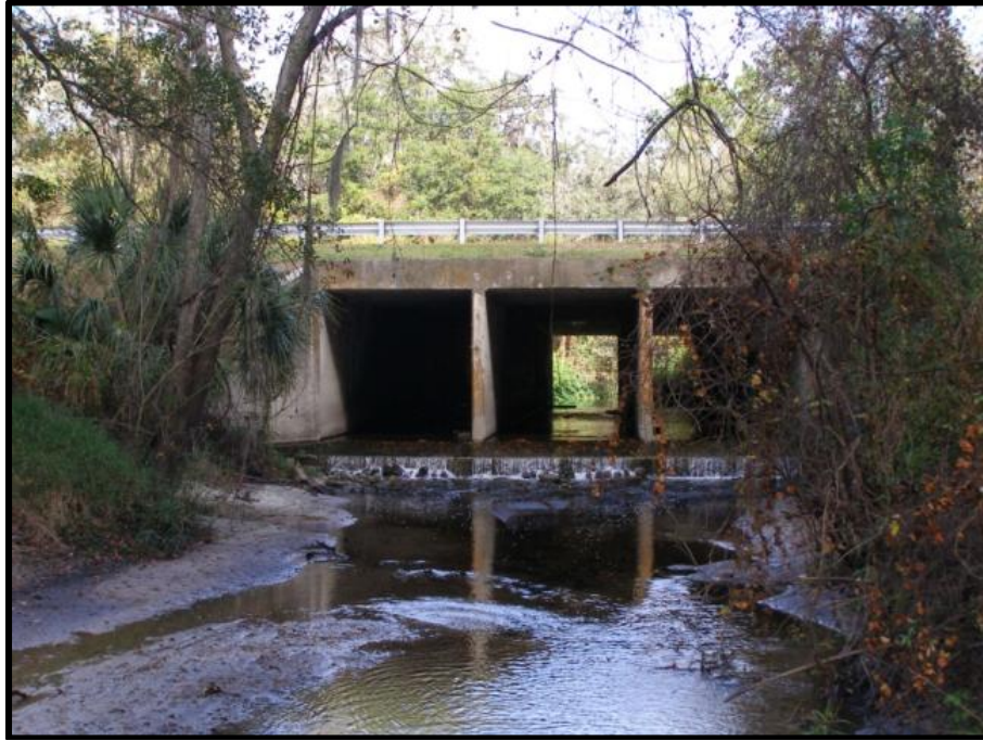
Photo 6-8. The south elevation of the Turkey Creek Culvert (FDOT No. 100058; 8HI11974).
