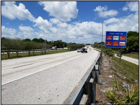
**Photo 4.** Southbound ROW conditions in the vicinity of 22<sup>nd</sup> Avenue. In this area of I-275, pavement widening and bridge widening will occur (see Sheet 12, **Appendix A**).
