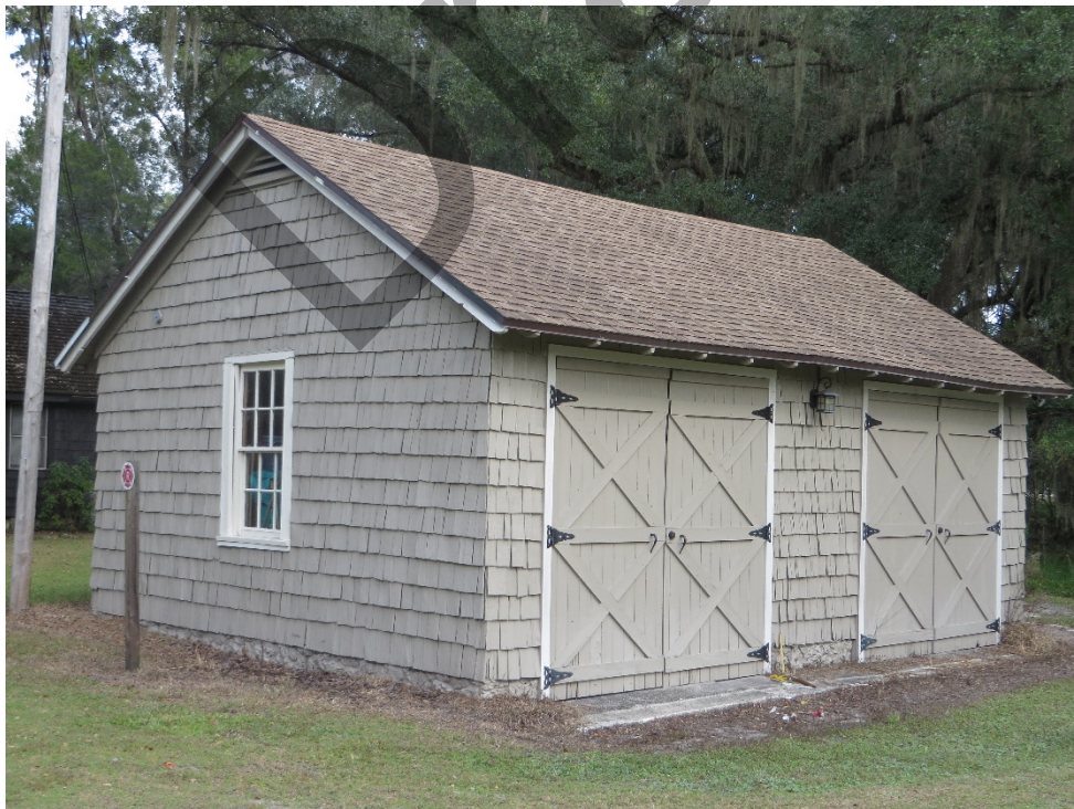
Photo 3. Maintenance Shed 2 (8HI03892), facing east.
