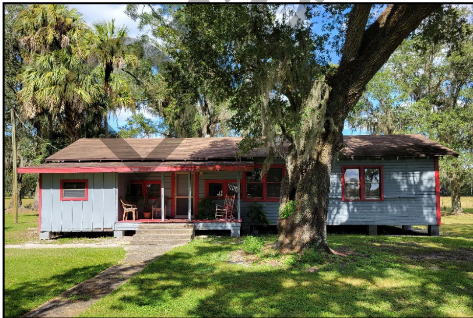
Photo 12. Road Camp No. 8502 - Building 1 (8HI15171), looking north-northeast.
