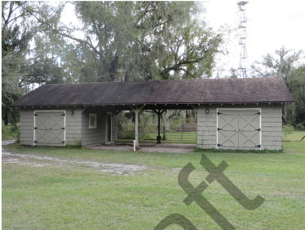
Photo 2. Maintenance Shed 1 (8HI03891), facing south.
