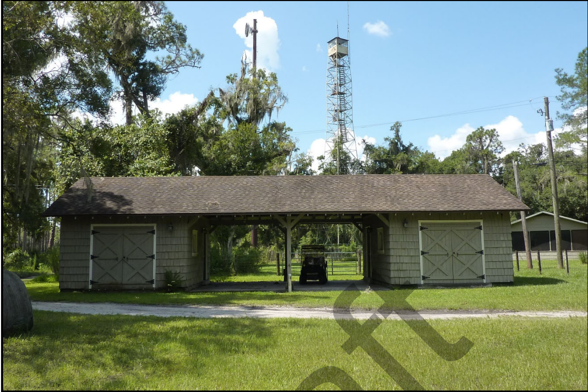
Photo 3. Maintenance Shed 1 (8HI03891), looking southwest.
