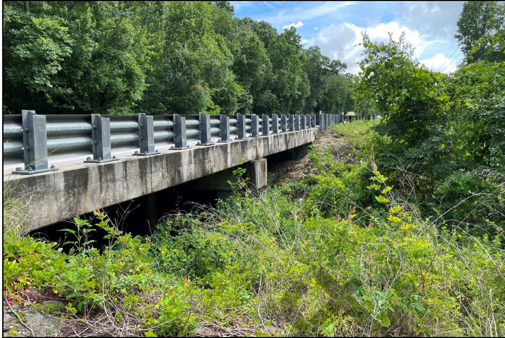
Photo 19. Photo 20. US 301 over Flint Creek relief (FDOT 100052) (8HI15446), looking northeast.
