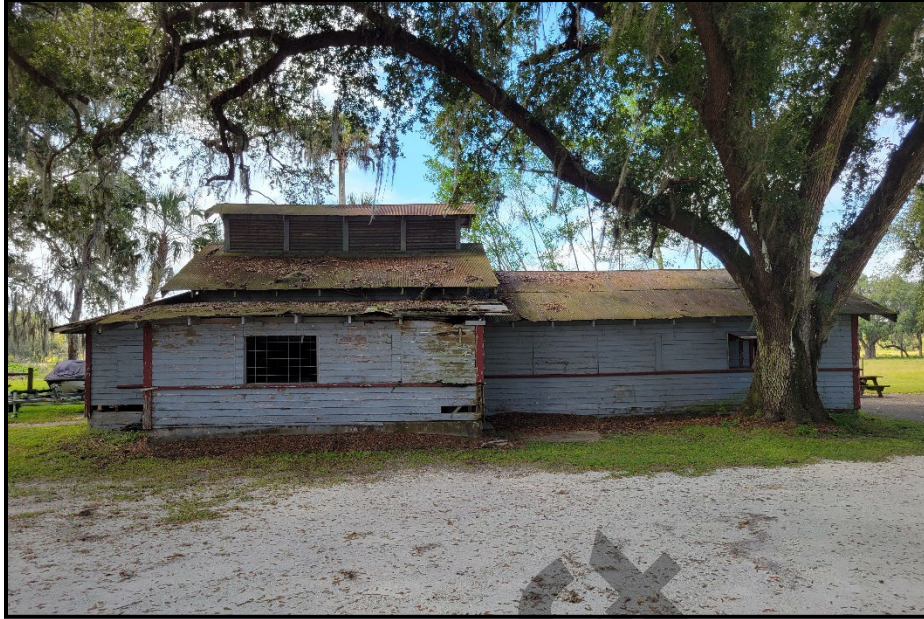
Photo 13. Road Camp No. 8502 - Mess Hall (8HI15172), looking northwest.
