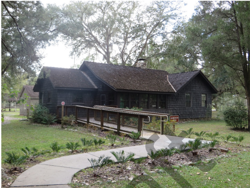
Photo 4. Ranger's Residence (8HI03893), facing east.
