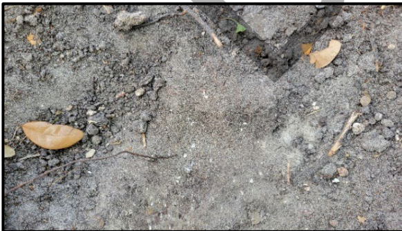
Photo 6. Limestone and gravel fill noted in SMF 3A.
