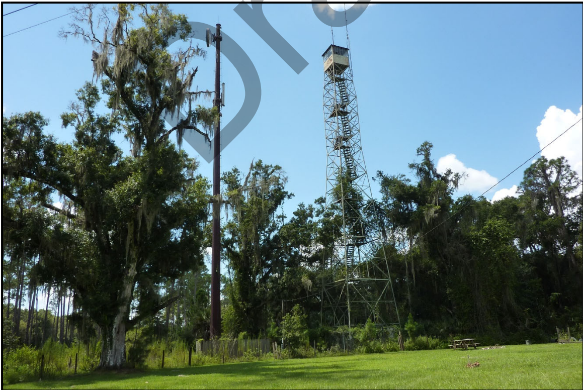
Photo 2. Fire Tower (8HI03890), looking southwest.
