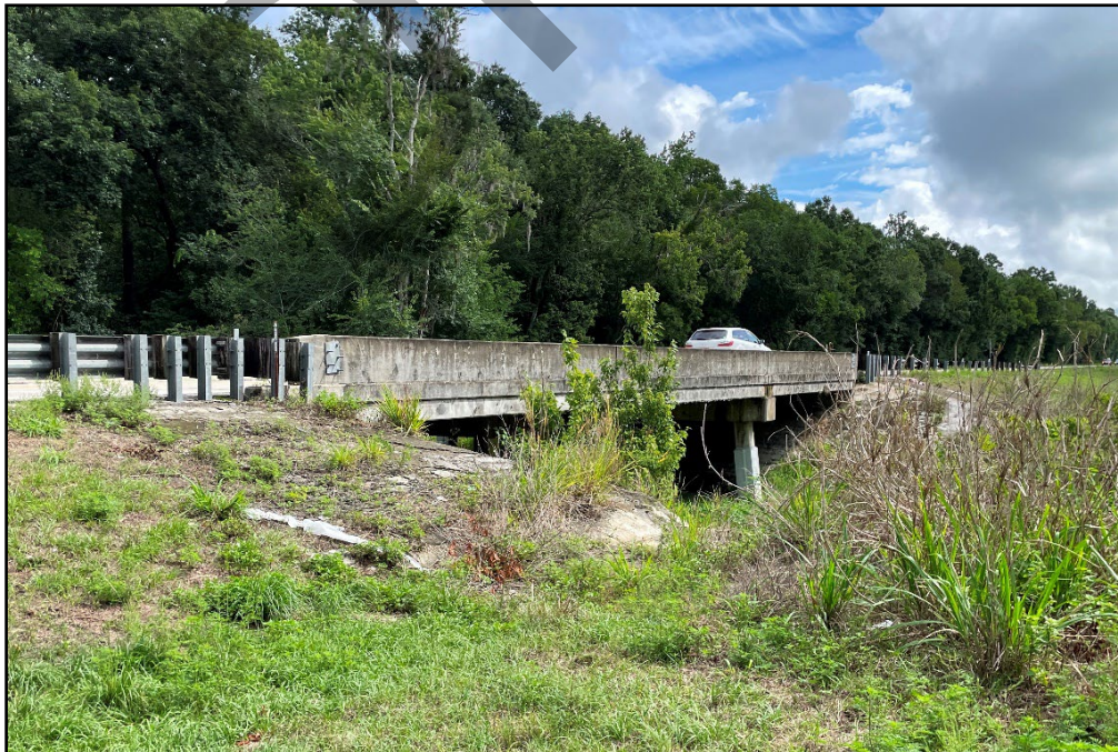
Photo 18. US 301 over Flint Creek (FDOT 100951) (8HI15445), looking north.
