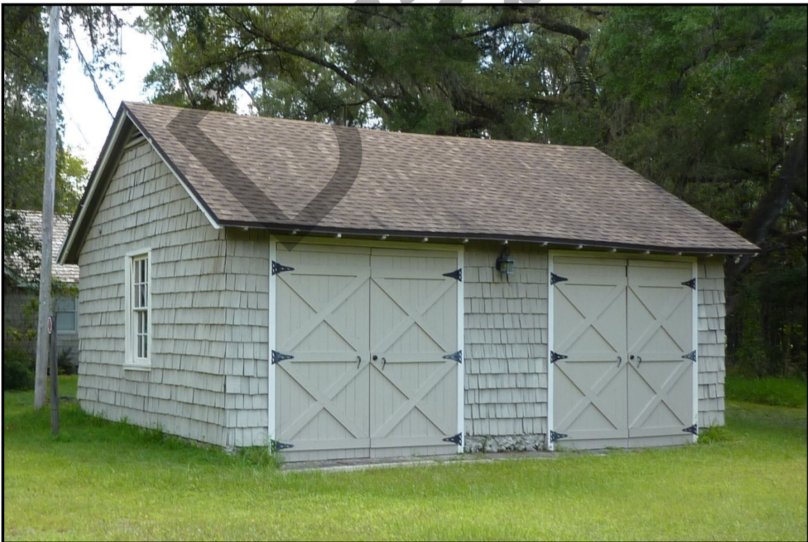
Photo 4. Maintenance Shed 2 (8HI03892), looking east.
