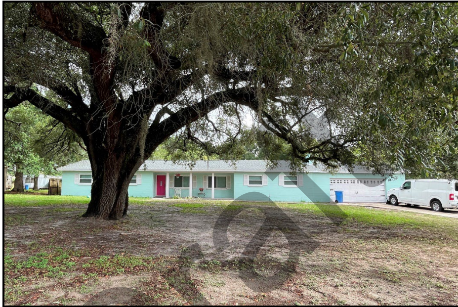
Photo 14. Masonry Vernacular style building (8HI15452) located at 9812 Rockhill Road, looking north.
