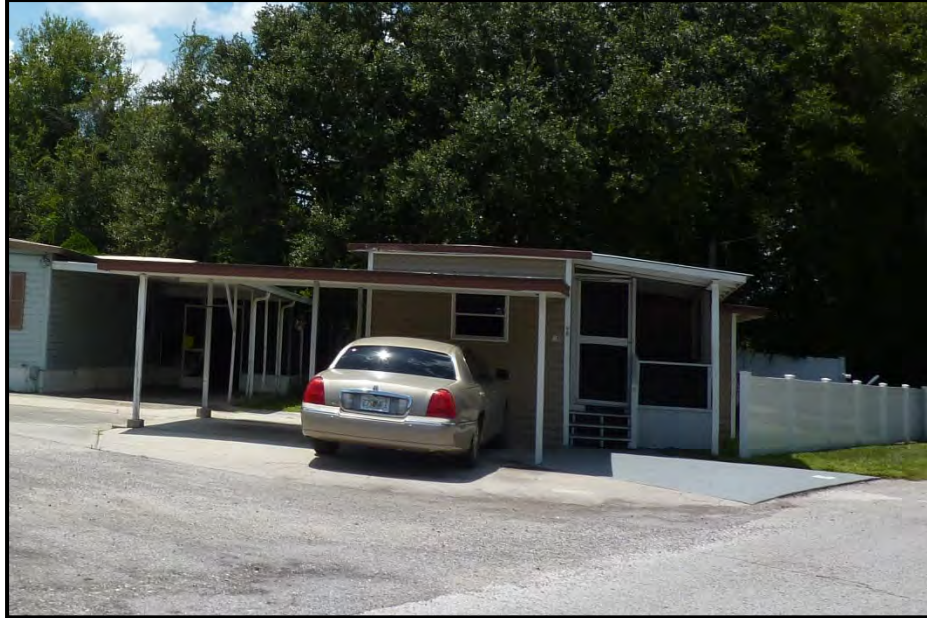
Photo 26. 11940 N US 301/Ranch Oaks Estates # 70 (8HI15146), looking southwest.
