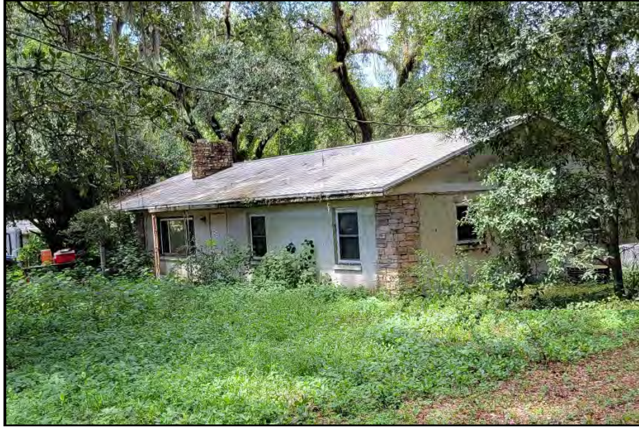
Photo 28. 13640 N US 301 (8HI15148), looking southwest.
