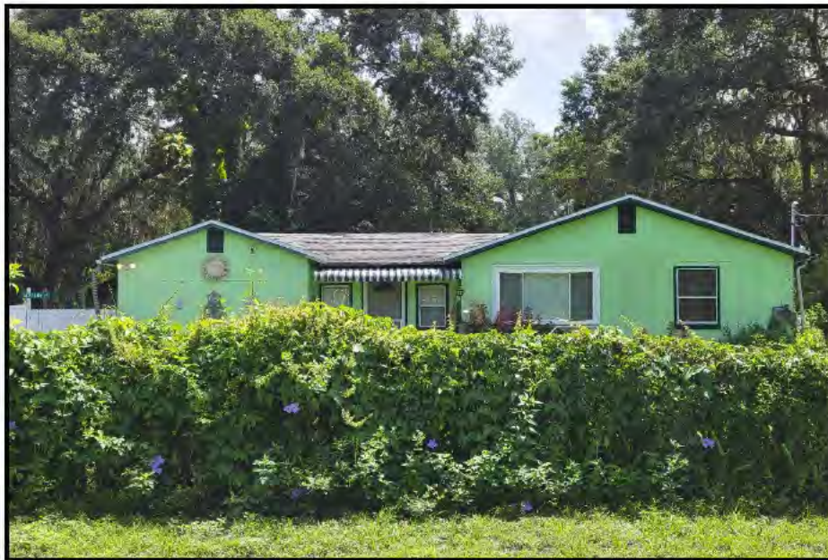
Photo 23. 12045 Jackson Road (8HI15143), looking east.
