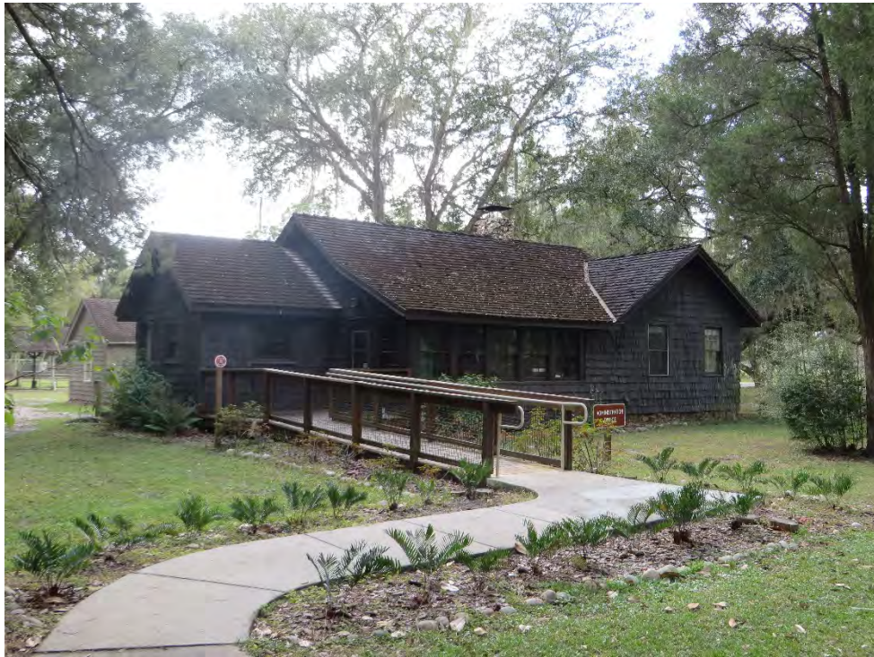
Photo 4. Ranger's Residence (8HI03893), facing east.
