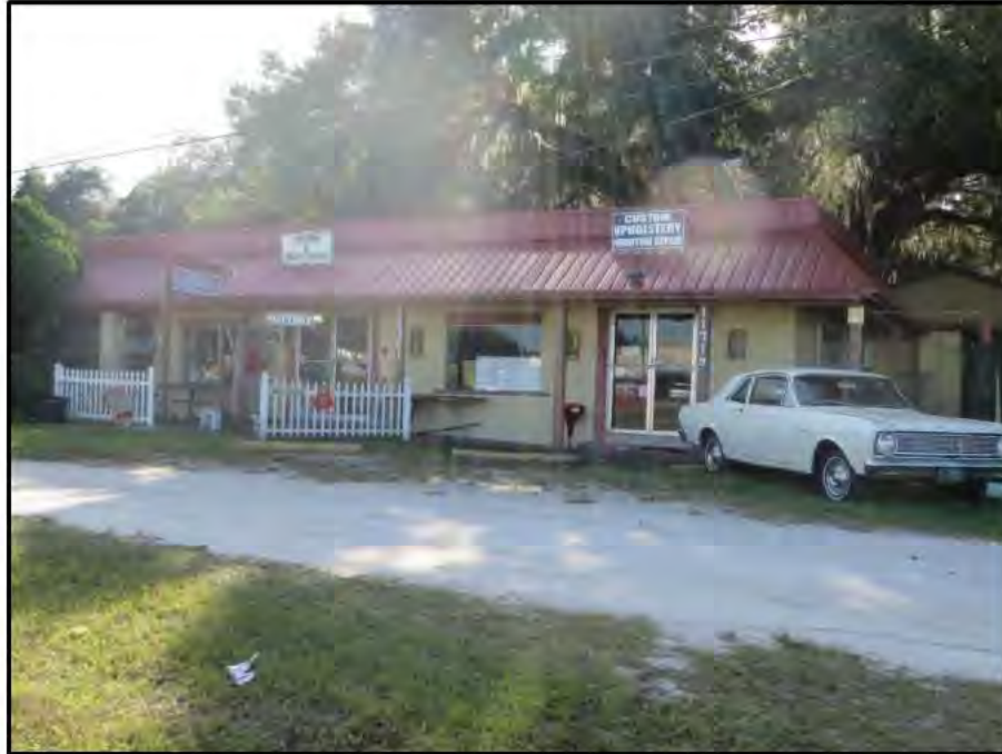
Photo 5.15: 11719 N. US Highway 301 (8HI13513), looking south
