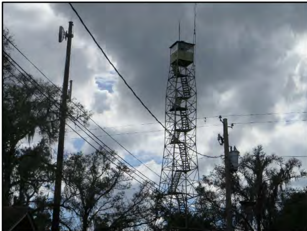
Photo 5.24. Fire Tower (8HI03890), looking southwest
