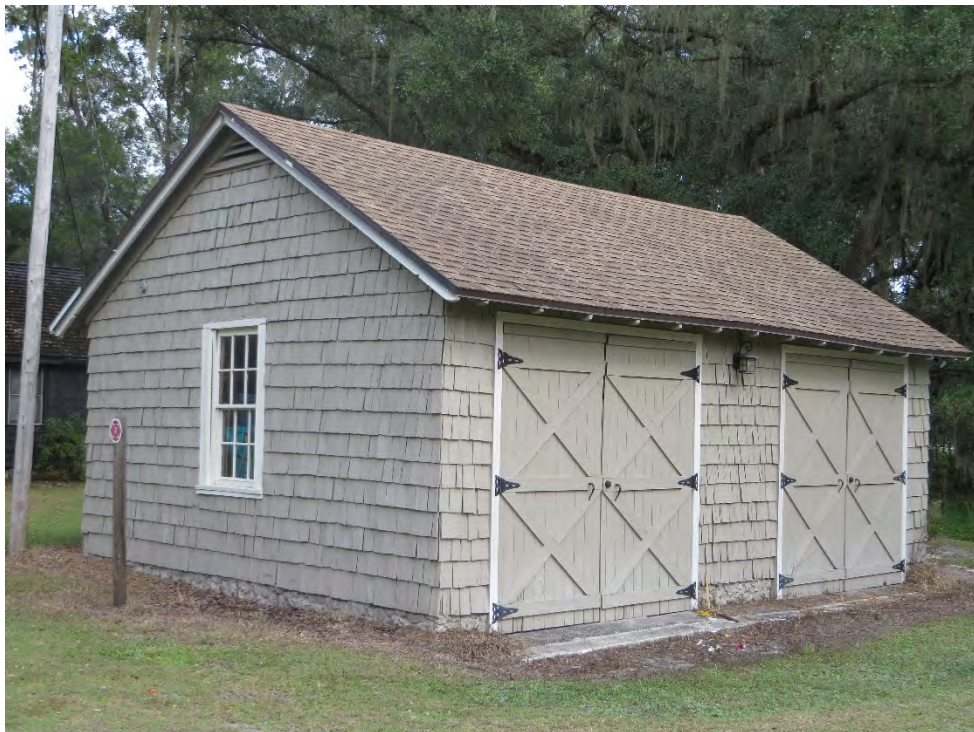
Photo 3. Maintenance Shed 2 (8HI03892), facing east.
