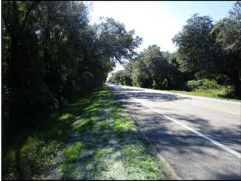
Photo 2.1: Looking southwest at forested area along the US 301 corridor
