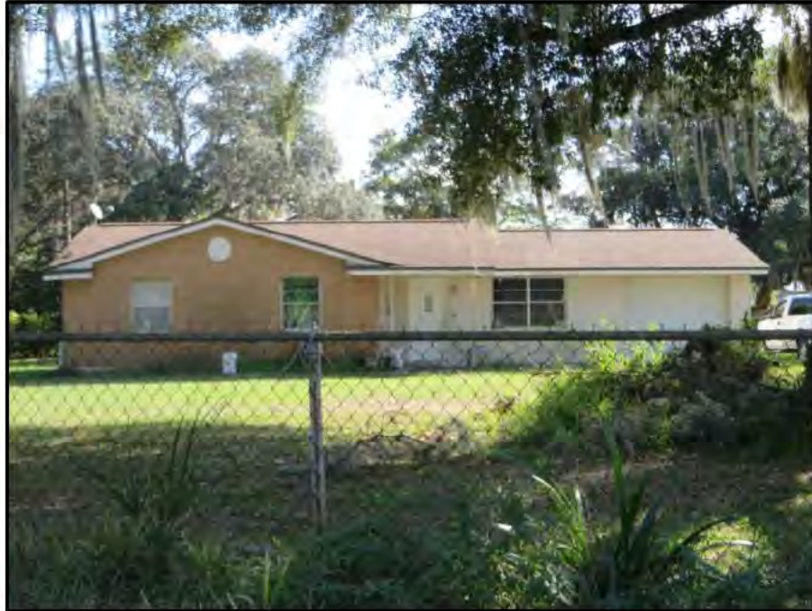
Photo 5.18: 11959 N. US Highway 301 (8HI13516), looking south
