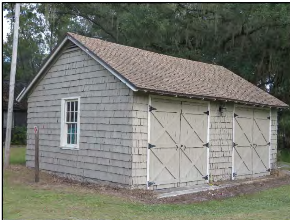
Photo 5.26. Maintenance Shed 2 (8HI03892), looking east
