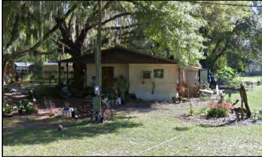
Photo 5.20: 14240 N. US Highway 301 (8HI13518), looking southwest
