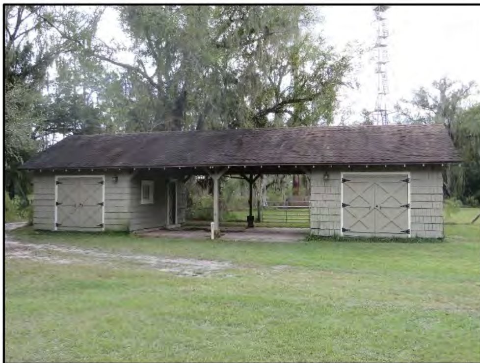
Photo 5.25. Maintenance Shed 1 (8HI03891), looking south
