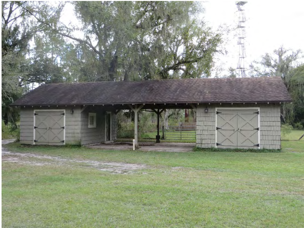
Photo 2. Maintenance Shed 1 (8HI03891), facing south.
