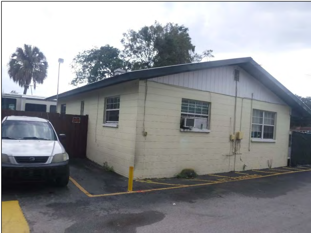
Figure 10-53 Glenwood Mobile Homes / 5001 Habersham Lane (8HI15323), Office Building, c. 1962, Considered National Register–Ineligible, Facing Southeast
