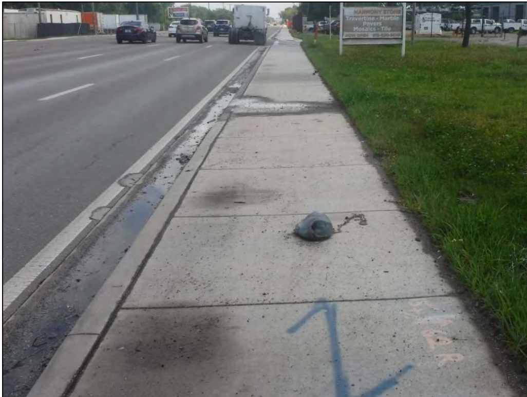
Figure 10-10 Representative View of Ditching and Hardscape Along US 41, Facing North Along US 41
