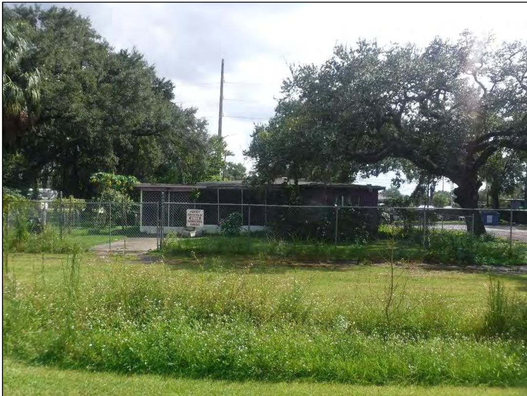
Figure 10-49 4711 El Camino Boulevard (8HI15336), c. 1959, Considered National Register–Ineligible, Facing South
