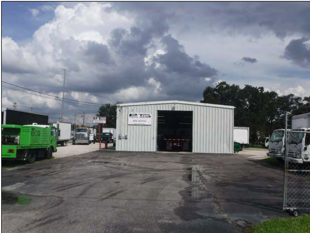
Figure 10-47 4901 Causeway Boulevard (8HI15334), c. 1973, Considered National Register–Ineligible, Facing East
