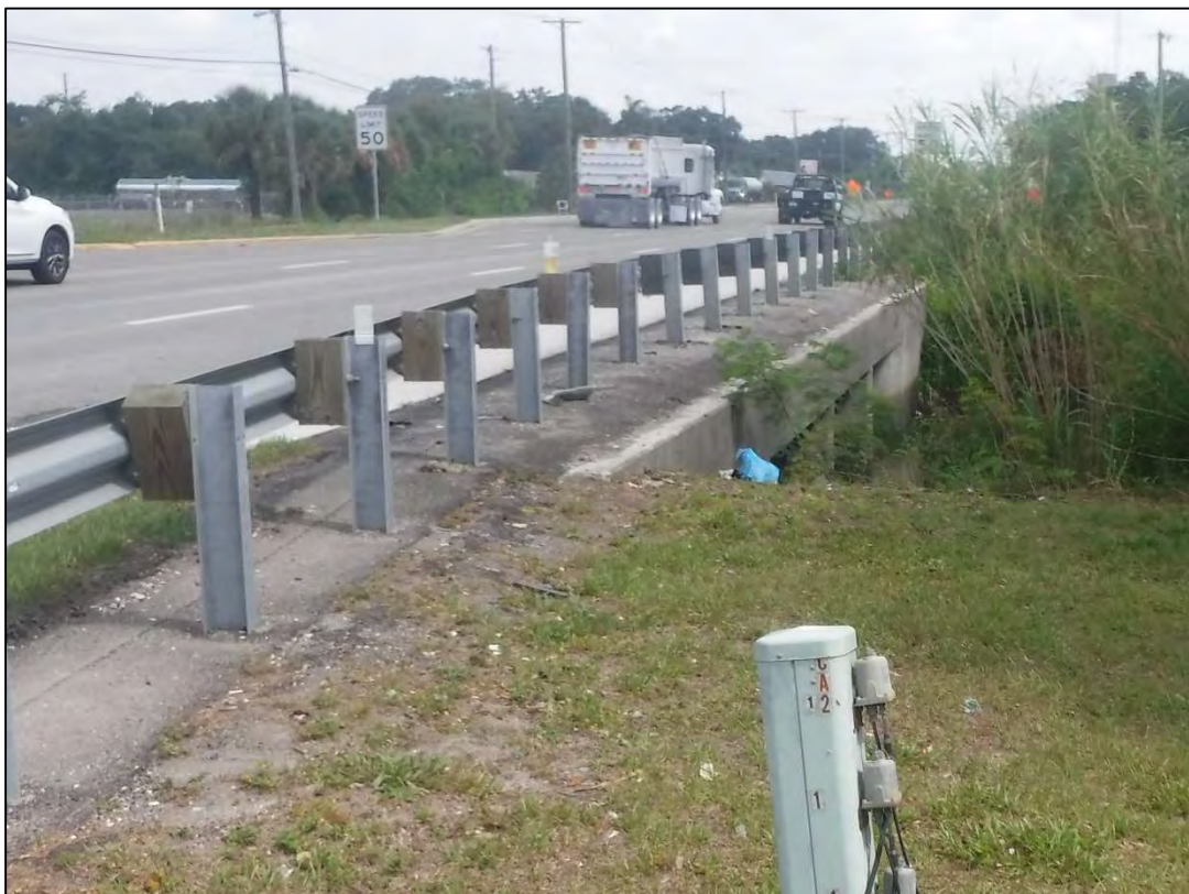
Figure 10-23 Delaney Creek (FDOT Bridge No. 100048) (8HI12023), Determined National Register–Ineligible, Facing North-Northwest
