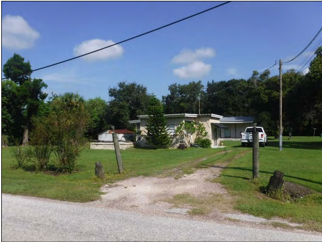
Figure 10-40 4710 Hartford Street (8HI15327), c. 1952, Considered National Register–Ineligible, Facing North-Northwest
