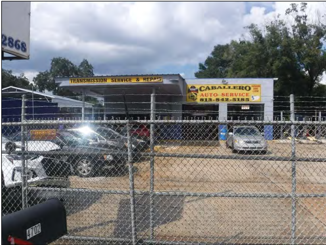
Figure 10-48 4702 E Causeway Boulevard (8HI15335), c. 1959, Considered National Register–Ineligible, Facing North
