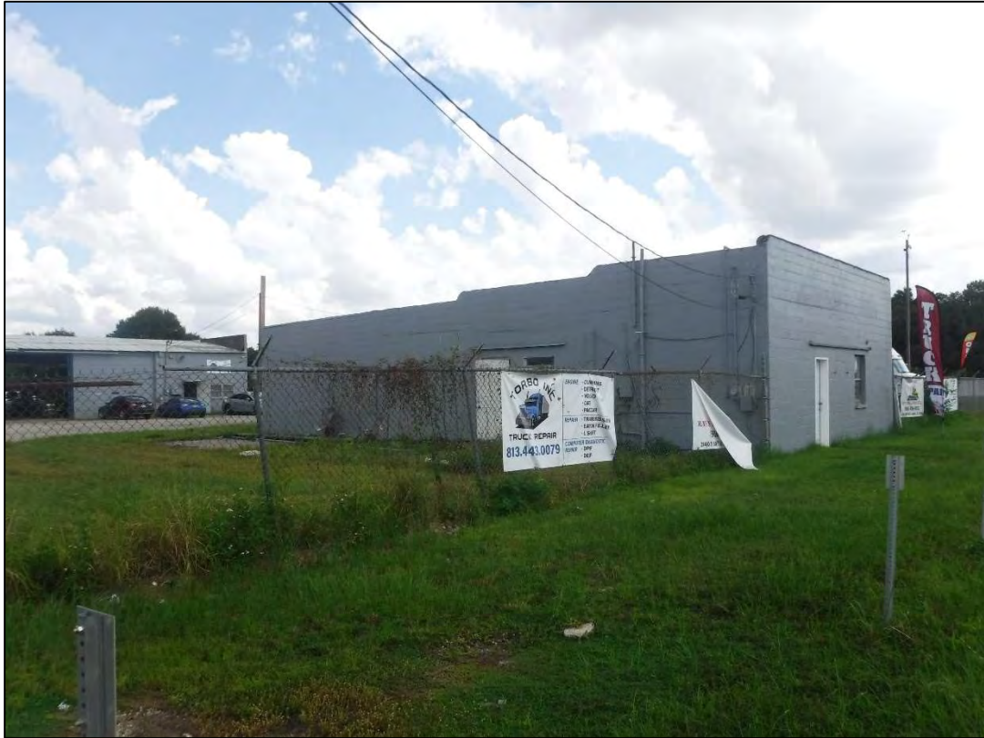
Figure 10-28 3140 S US 41 (8HI12109), Determined National Register–Ineligible, Facing Southeast
