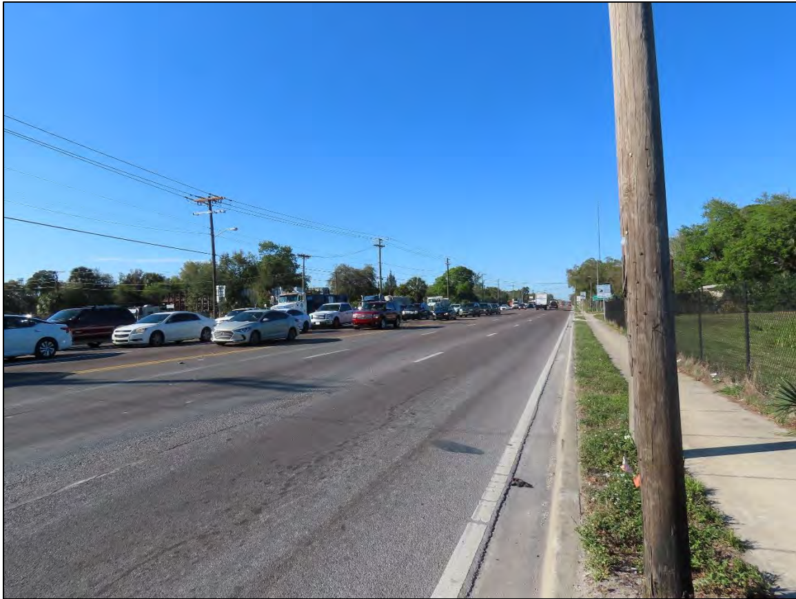
Figure 1: US 41 (8HI12129), c. 1915, considered National Register–ineligible, facing North
