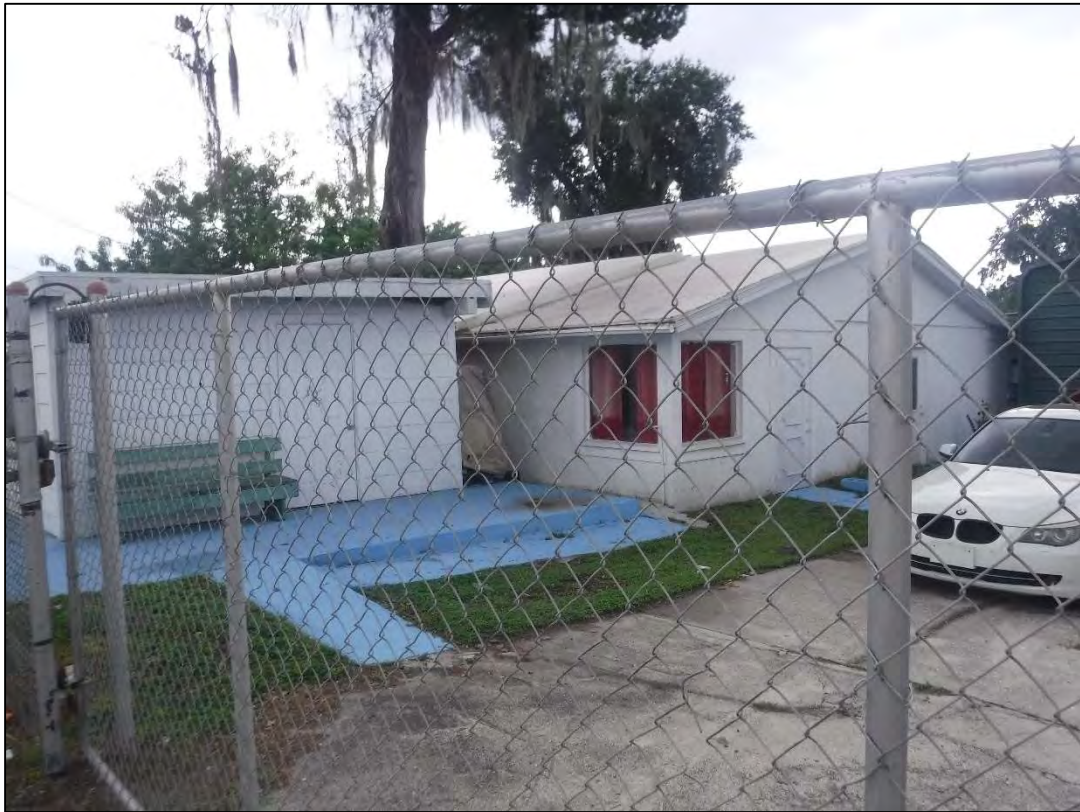
Figure 10-52 2319 S 50 th Street (8HI15339), c. 1951, Considered National Register–Ineligible, Facing Southwest
