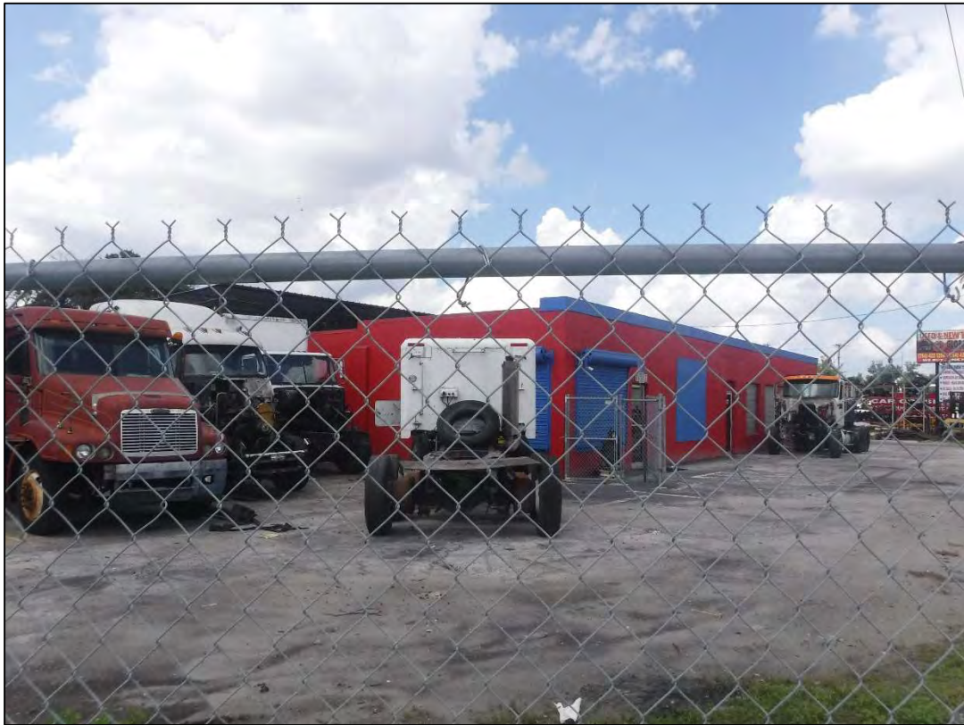
Figure 10-30 2923 S US 41 (8HI12111), Determined National Register–Ineligible, Facing Northwest
