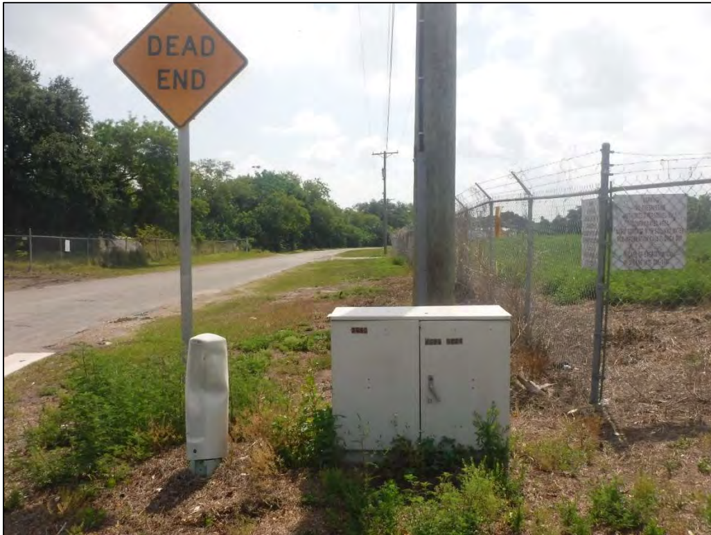
Figure 10-12 Representative View of Underground Utilities and Hardscape Preventing Testing Along US 41, and Sign Designating Contaminated Soils, Facing East
