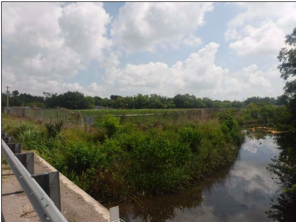
Figure 10-13 View of Lot Containing Contaminated Soils along Delaney Creek, Facing Northeast
