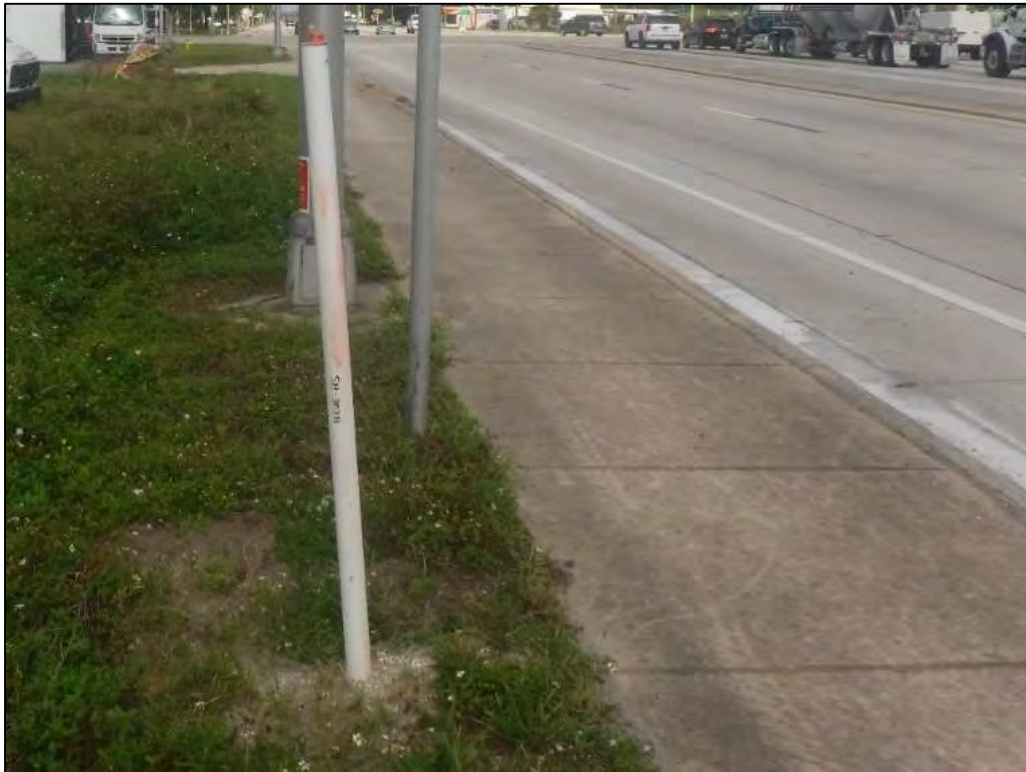
Figure 10-16 Representative View of Indicators of Underground Utilities and Hardscape Preventing Testing Along US 41, Facing North Along US 41
