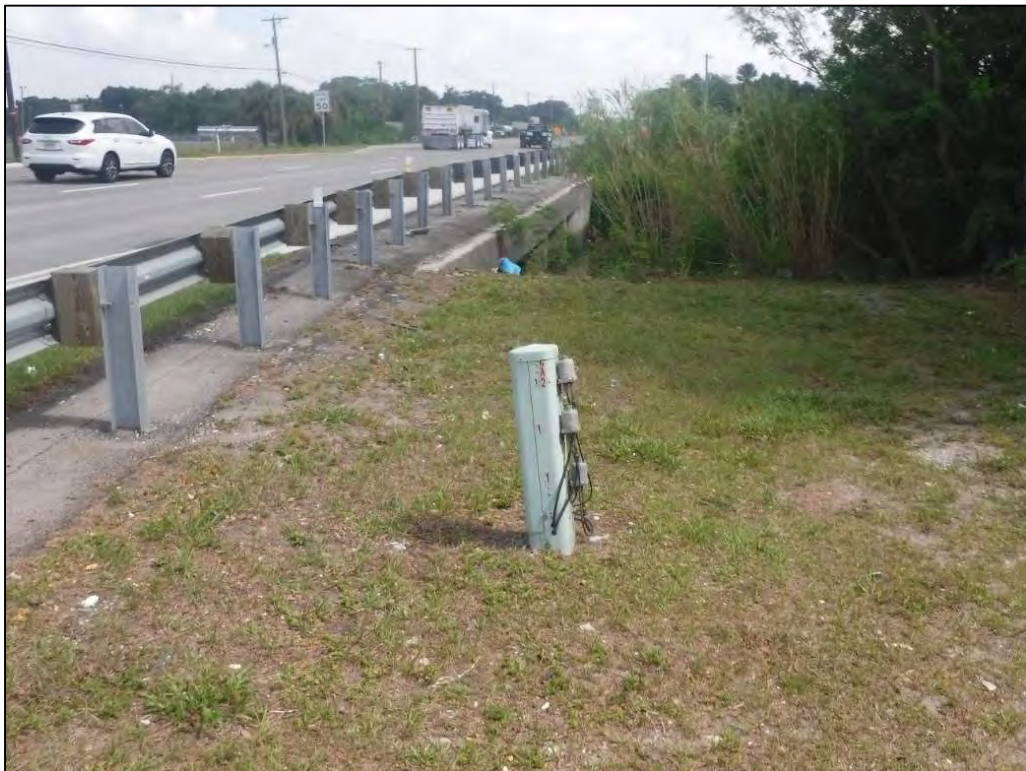
Figure 10-11 Representative View of Indicators of Underground Utilities, Hardscape, and Creek Preventing Testing Along US 41, Facing North Along US 41 Towards Delaney Creek
