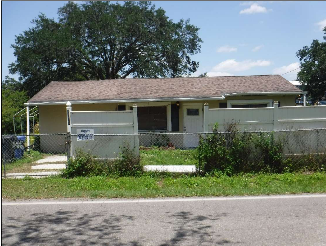
Figure 10-11: 5016 Hartford Street (8HI15402), Considered National Register-Ineligible, facing North
