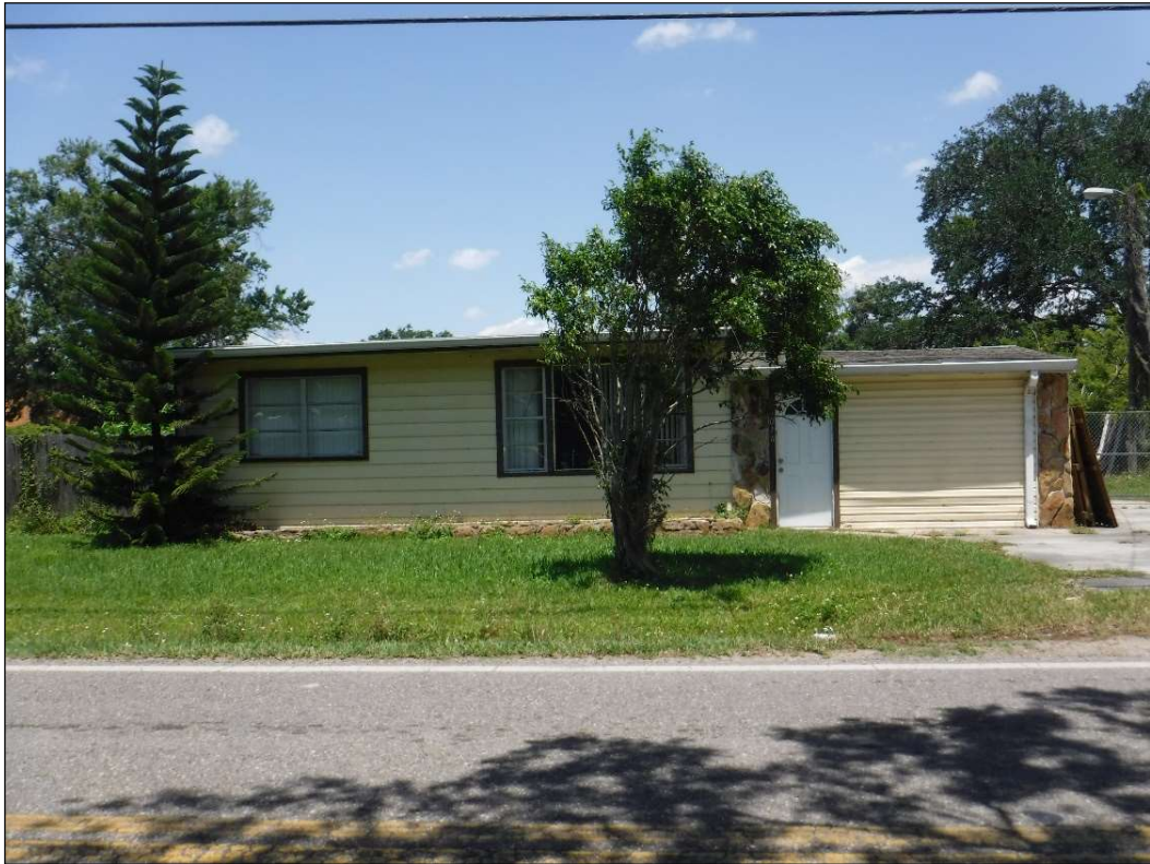
Figure 10-10: 5014 Hartford Street (8HI15401), Considered National Register-Ineligible, facing North
