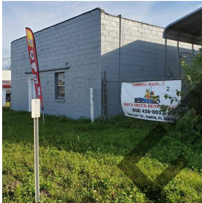
Site 21 – Torbo Truck Repair (former Southeast Industrial) West boundary looking northeast
