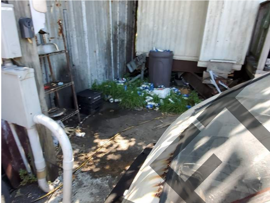
Site 66 – Garage On Wheels Stained soil and concrete along north-central boundary, looking northeast at office trailer
