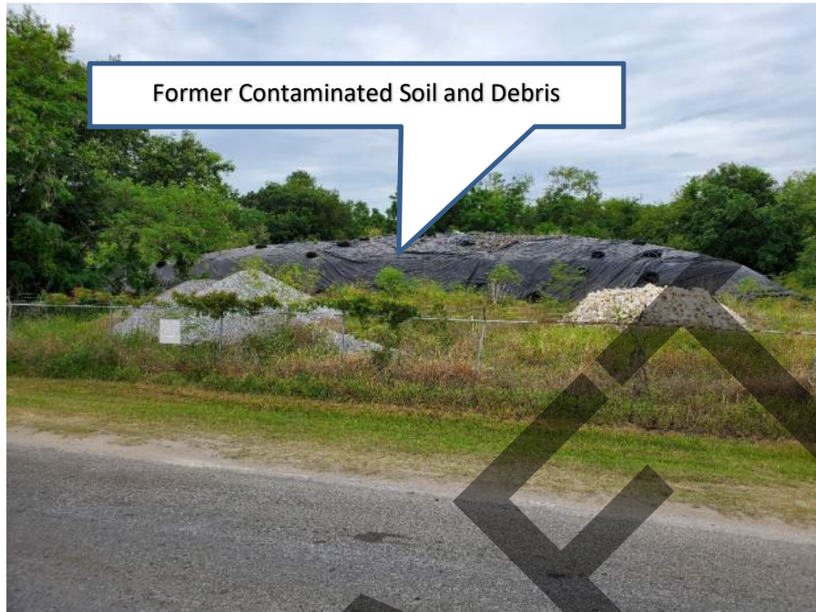
Site 14/15/16/17 – Exide Technologies/Delaney Creek Brownfield Redevelopment Area East of US 41 looking northwest, south of 36 th Avenue South
