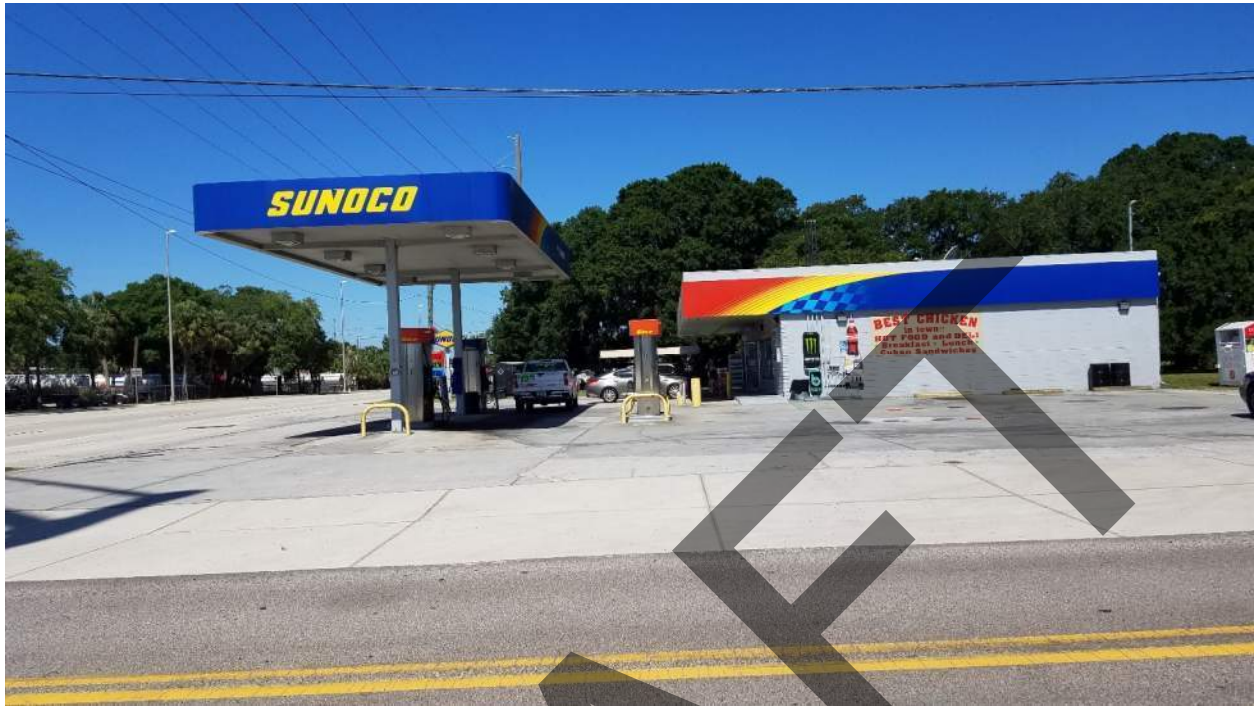
Site 33 – Sunoco (Former United Oil #215) East boundary looking west
