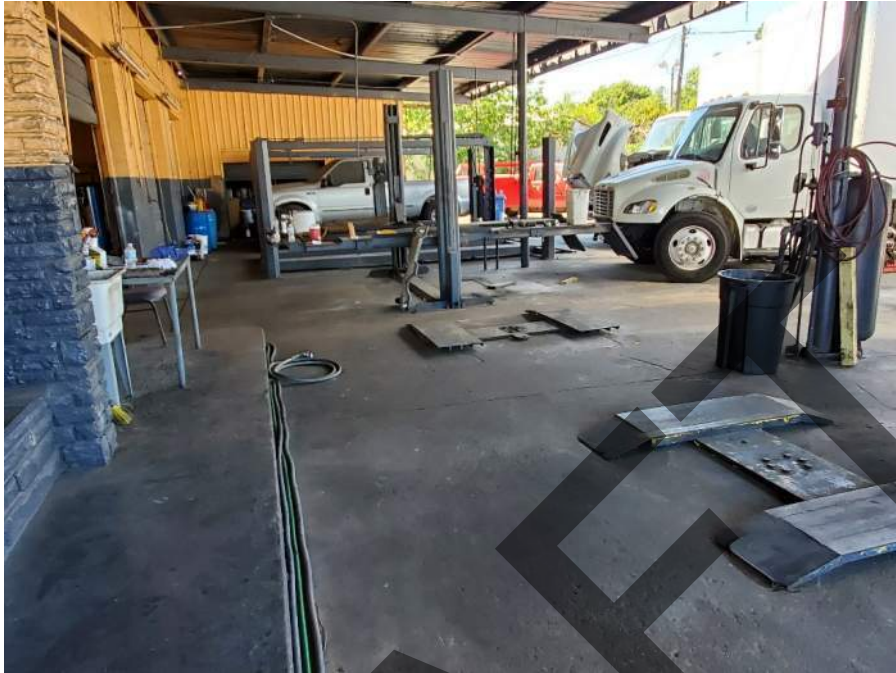
Site 67 – Avengers Auto Body/DMD Motors (former CSD Truck Repairs) Service bays with hydraulic lifts
