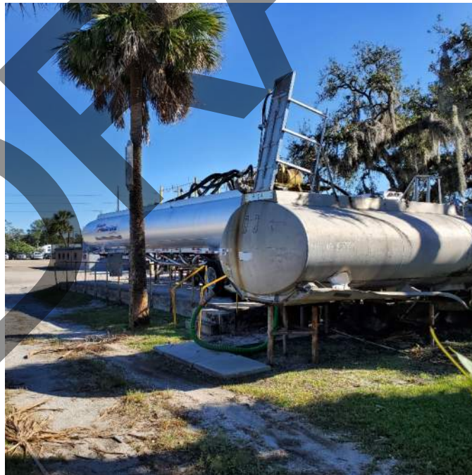
Site 28 – Florida Tank Services (formerly Talman Tank and Equipment) West boundary looking southeast at tanker pumping area
