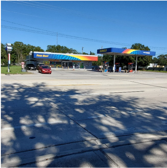
POND 3B – East parcel South of Sunoco looking north
