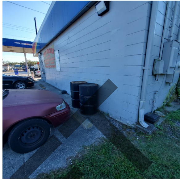
POND 3B – East parcel Northeast corner of building looking south
