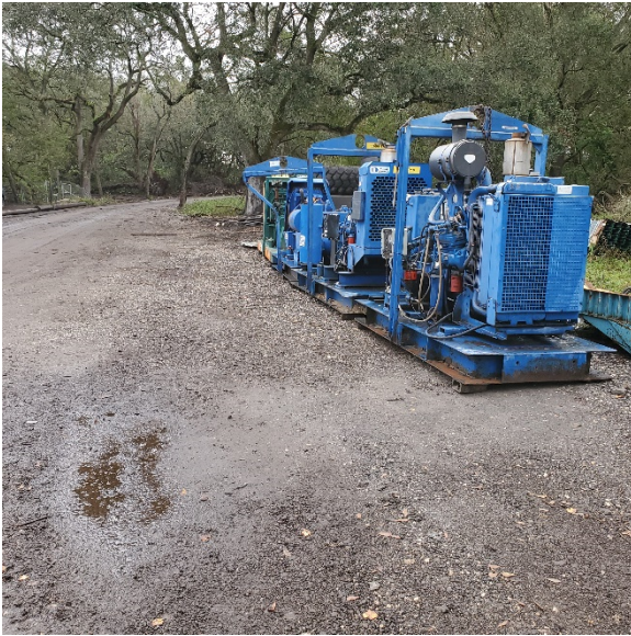
POND 2B – Dewatering pumps, east-central area looking east
