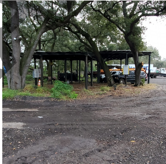
POND 2B – Shed in northwest area West of shed looking east
