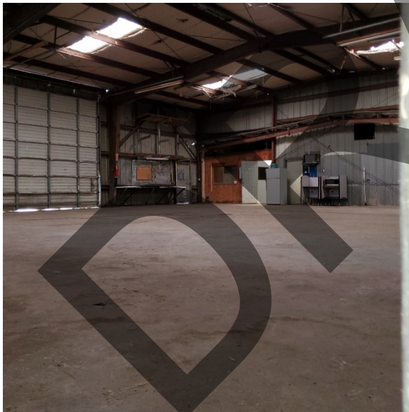
POND 1A – inside building looking northeast
