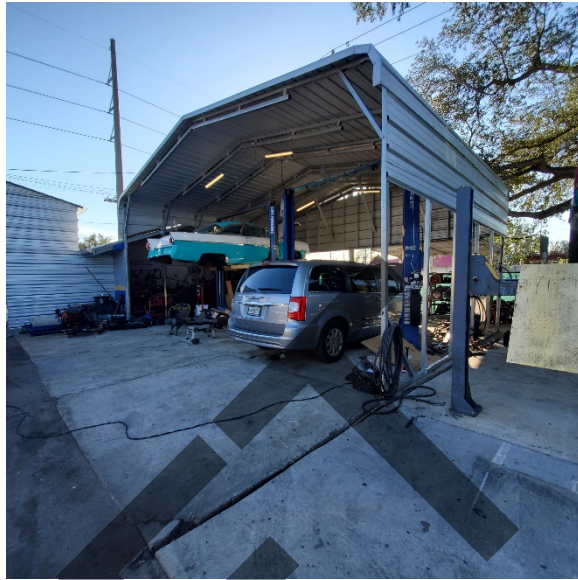
POND 3B – R&E Tire Plus (West parcel) Northeast central area looking southwest
