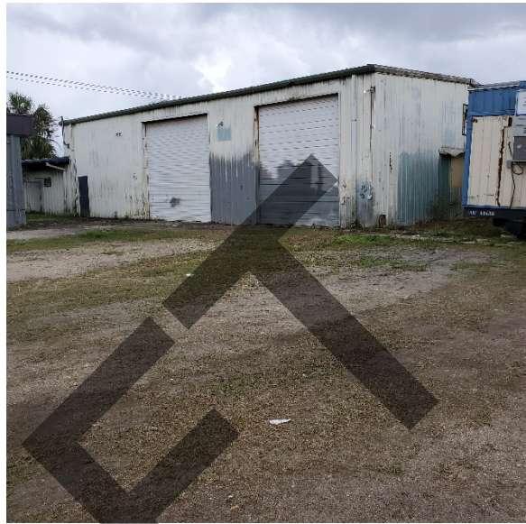
POND 1A – Vacant building East-central area looking southeast
