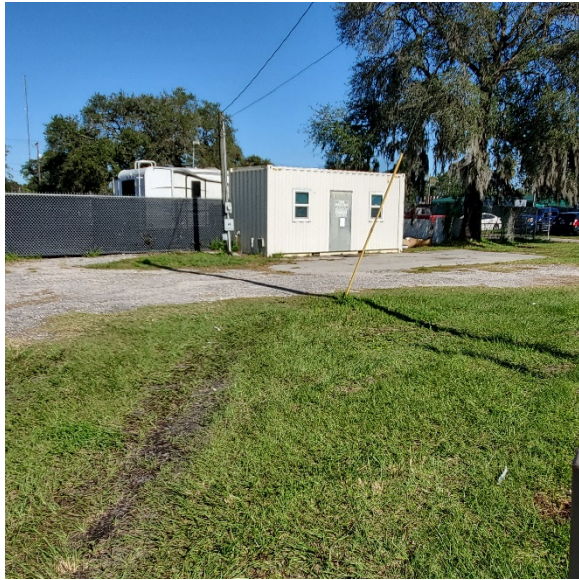
POND 3A - West parcel, First Choice Cars (4902 Causeway Blvd) Near south boundary looking northeast
